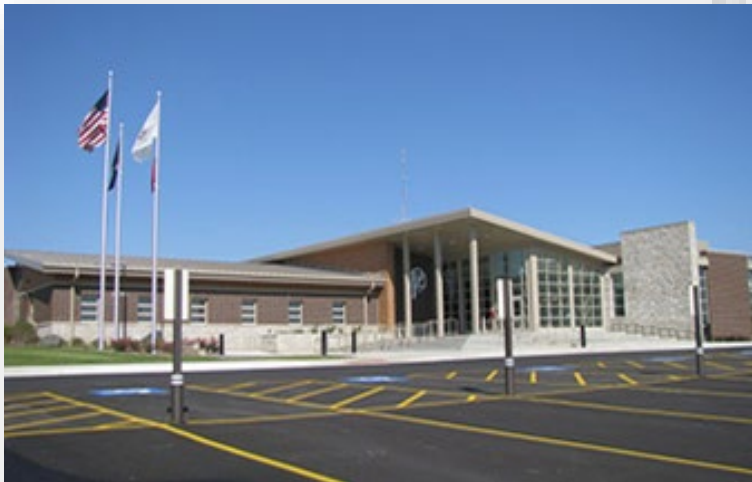
PFPD Administration Campus
